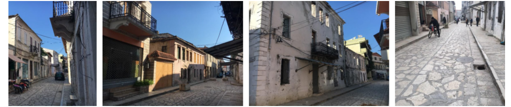
Fig. 3. Pre-intervention condition along Justin Godard Street. Source: Atelier 4.
